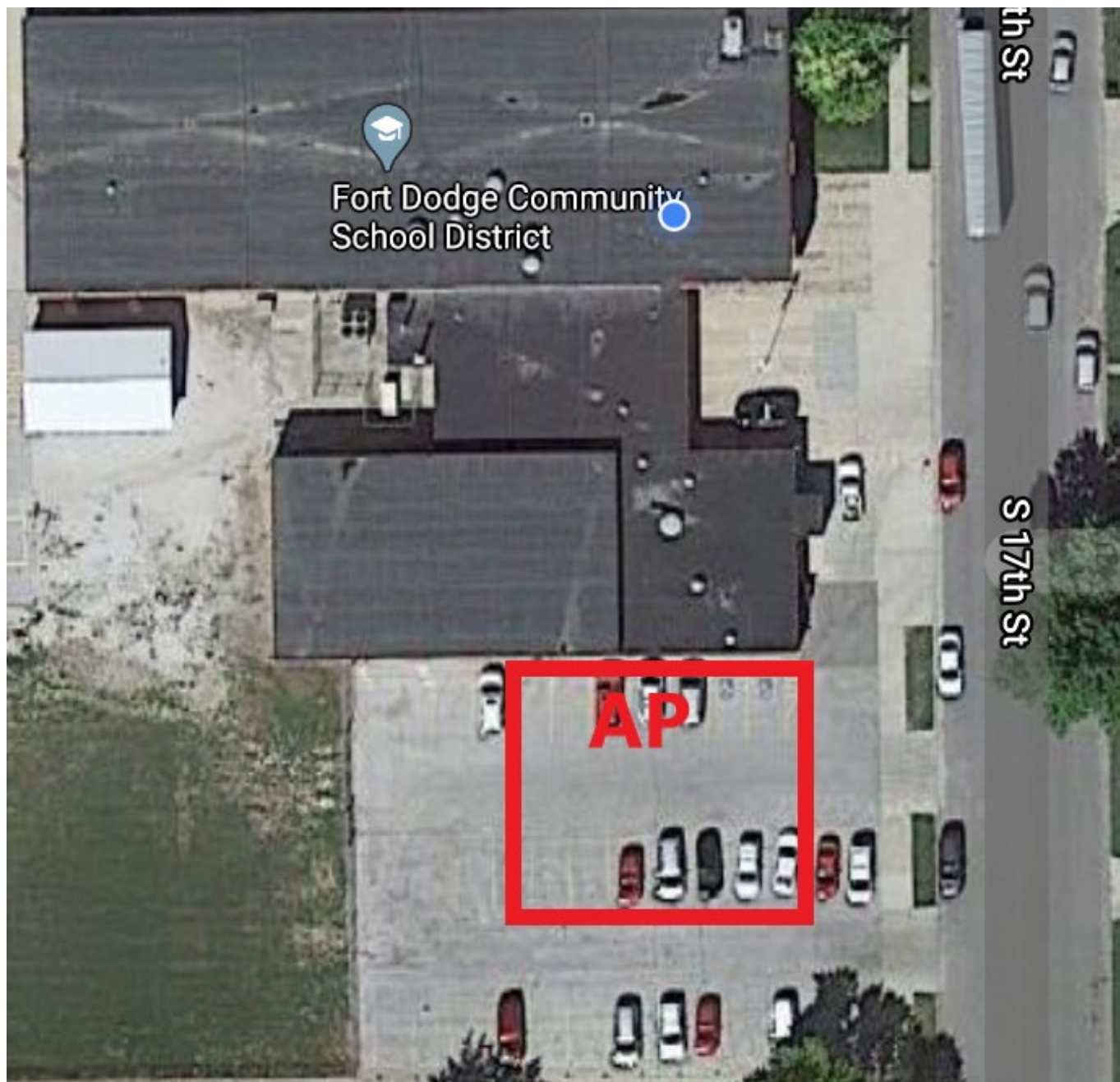
CENTRAL OFFICE (south side of building)
